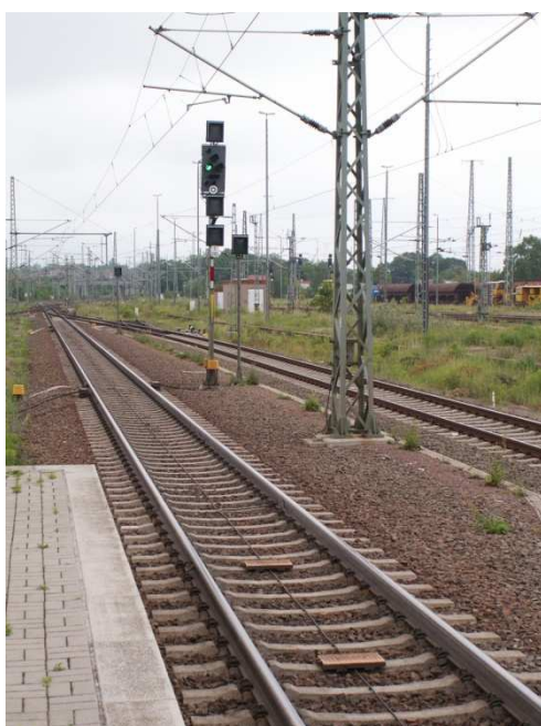
ETCS-beacon on a German track.
